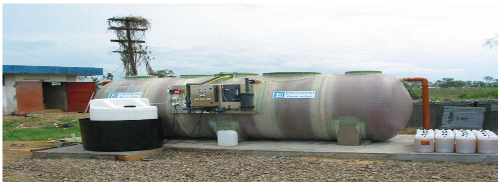
Picture 6.1 The Swedish UN-forces treatment plant in Liberia, this plant is for 230 persons.
