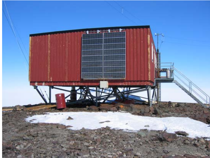
Figure 10: Solar panels at Wasa station Source: Swedish Polar Research Secretariat
